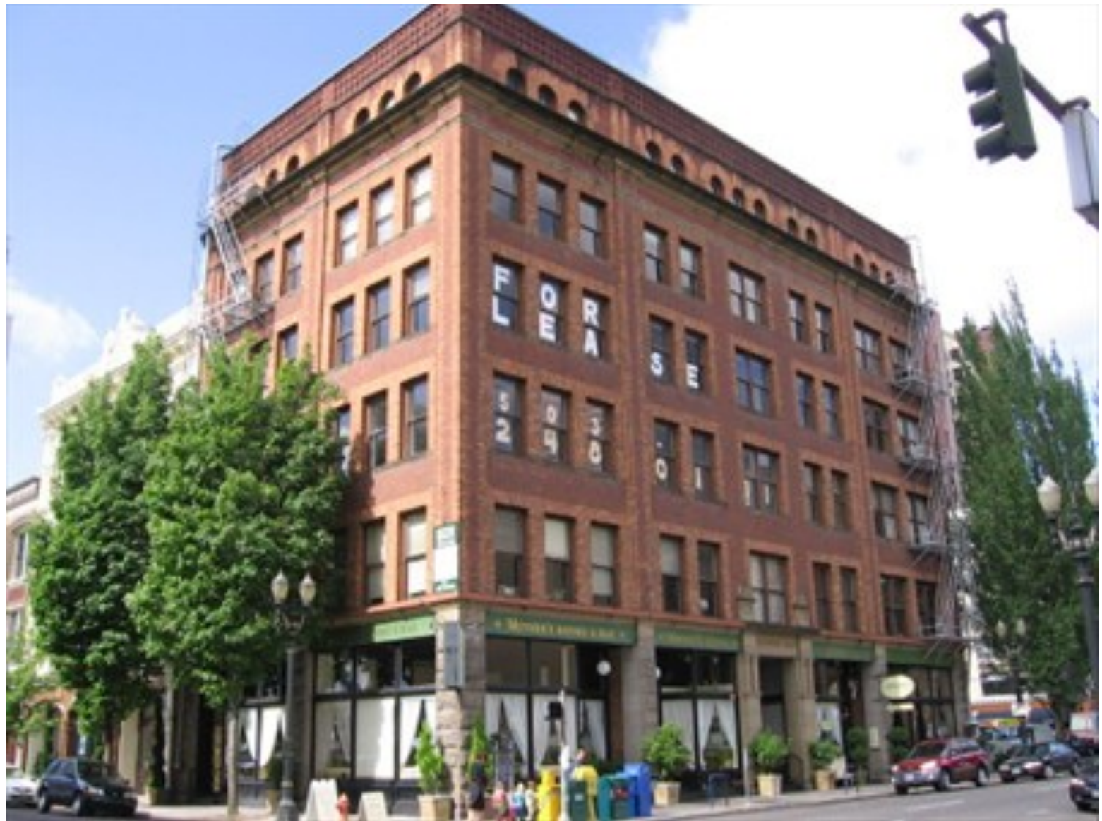
Concord Bldg, SW 2 nd and Stark 1891 William S Ladd and Sons
