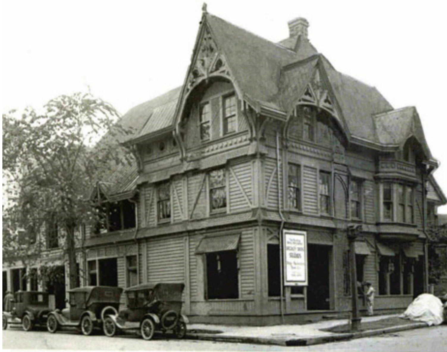
Ladd Carriage House 1927
